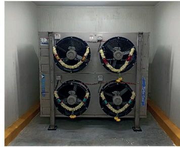
FLOOR MOUNTED BLAST FREEZER EVAPORATOR
